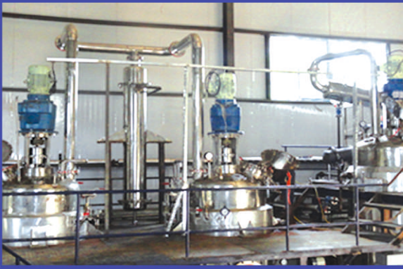
Natural Colours Extraction Plant
